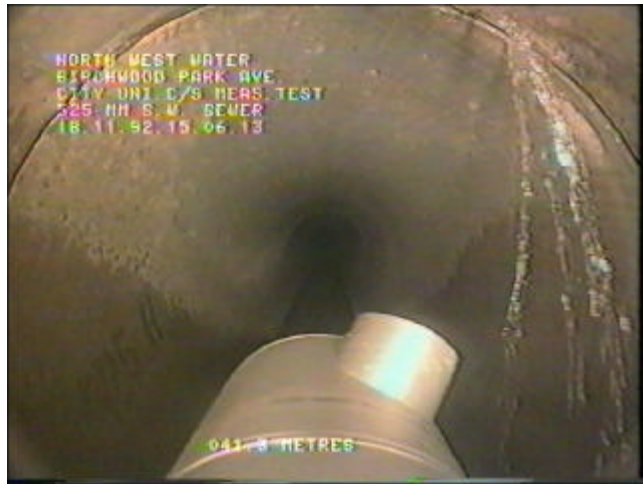
Fig. 12. An image of the profiler in the sewer.
